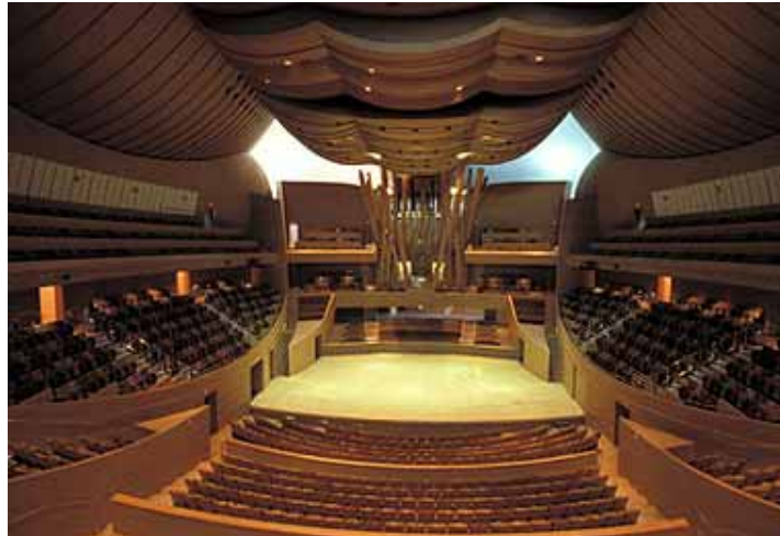
Eighty four curved structures, each containing about 80 panels, form the ceiling of the Walt Disney Concert Hall at the Music Center of Los Angeles County.
